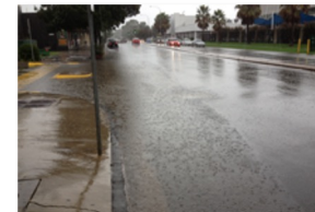
Flooding / surface water
